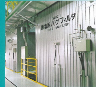
集じん用バグフィルタ(左)と 脱塩用バグフィルタ(右) NO.1 Bagfilter (left) and NO.2 Bagfilter (right)
